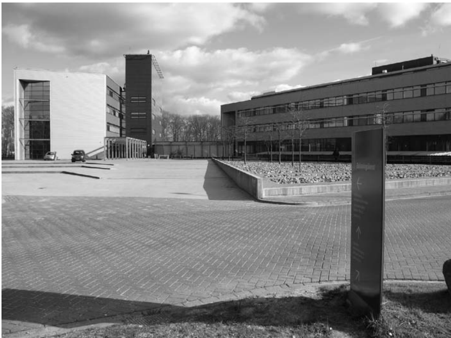
Plate 1. Exterior of the building of the case organization
